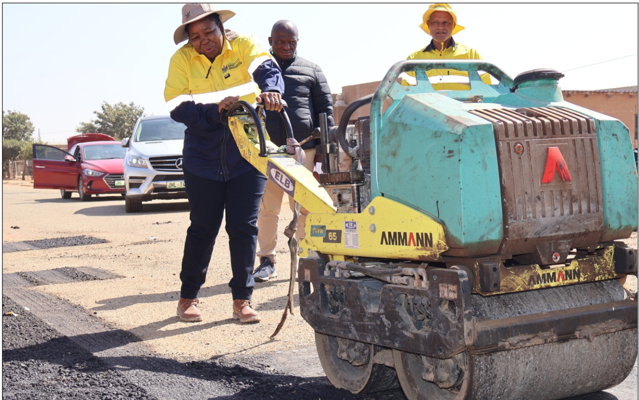
MEC Sempe Elizabeth Mokua during Thuntsha-Lerole Accelerated Service Delivery Programme in Biesiesvlei in Ditsobotla Local Municipality. The departmental roads maintenance team patching potholes on several internal roads in the community. MEC Mokua is seen operating a Hydrostatic Drive Roller Hand Roller Compactor
